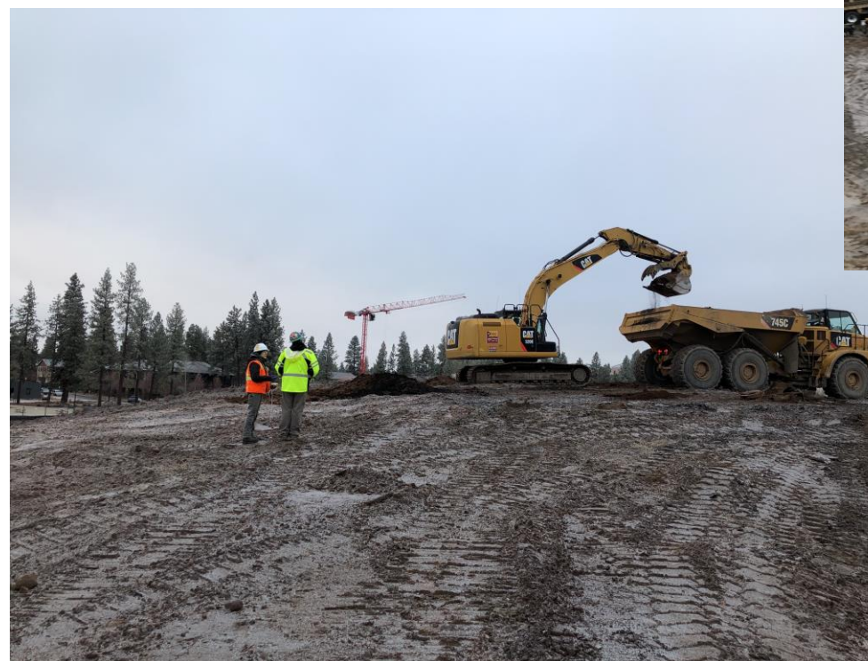
Cell 2 Top Soil work
