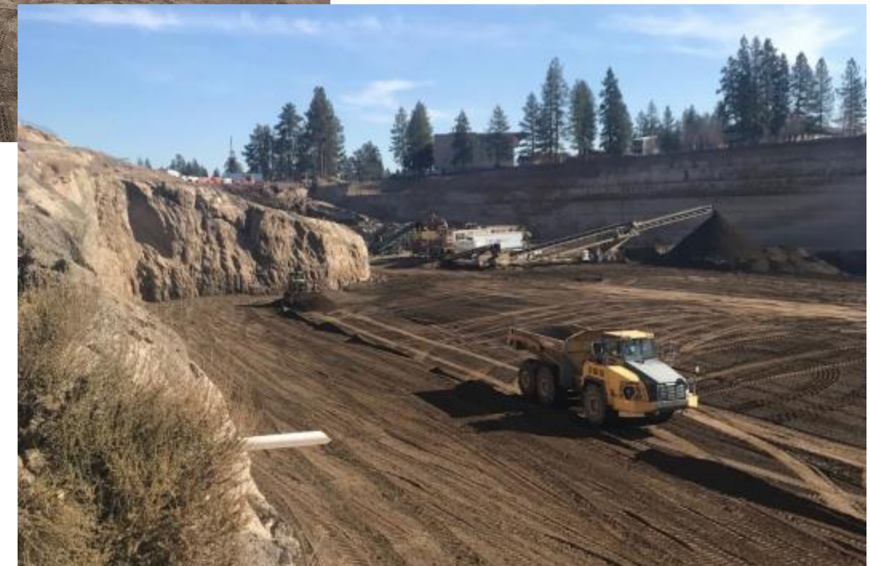
North side of pit activities
