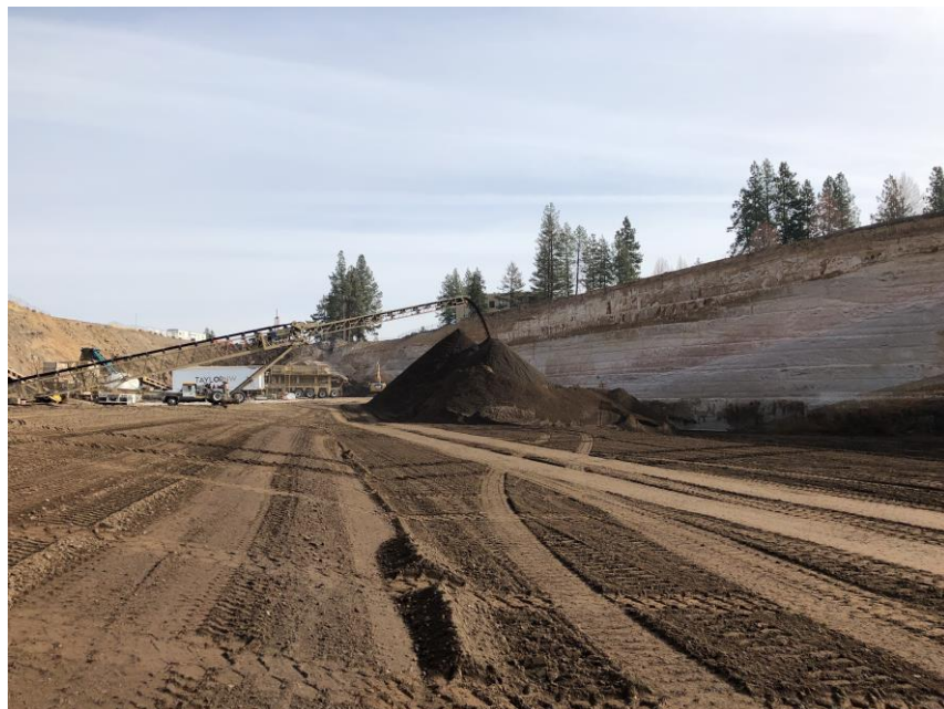
Crusher Stockpile and South Benching
