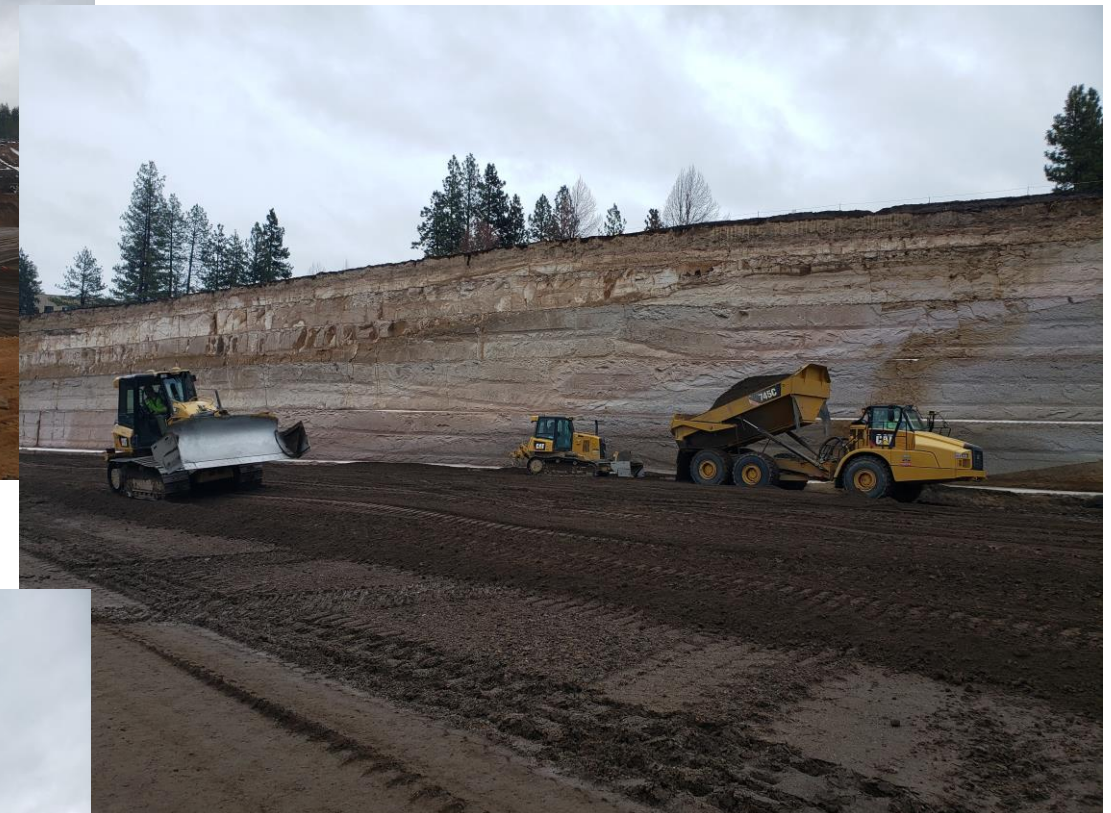
Filling Pit Floor Continued
