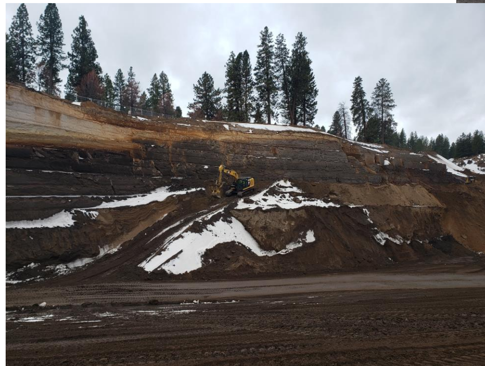
Southwest Benching activities ongoing
