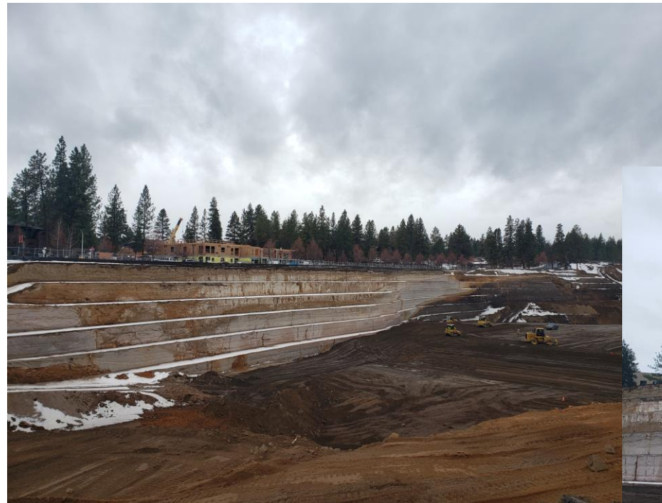
South Side of Pit benching and filling pit floor activities
