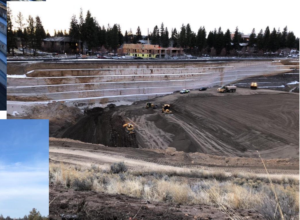
Filling Pit Floor Continued
