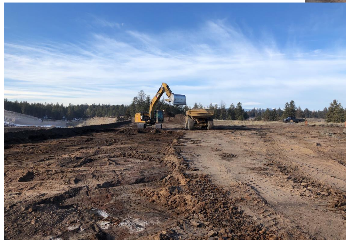
Cell 2 clearing, grubbing, and top soil work
