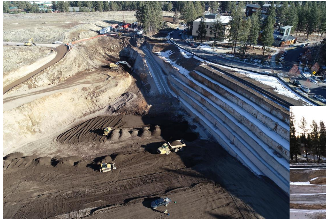
Aerial View of South Side of Pit benching and filling pit floor activities
