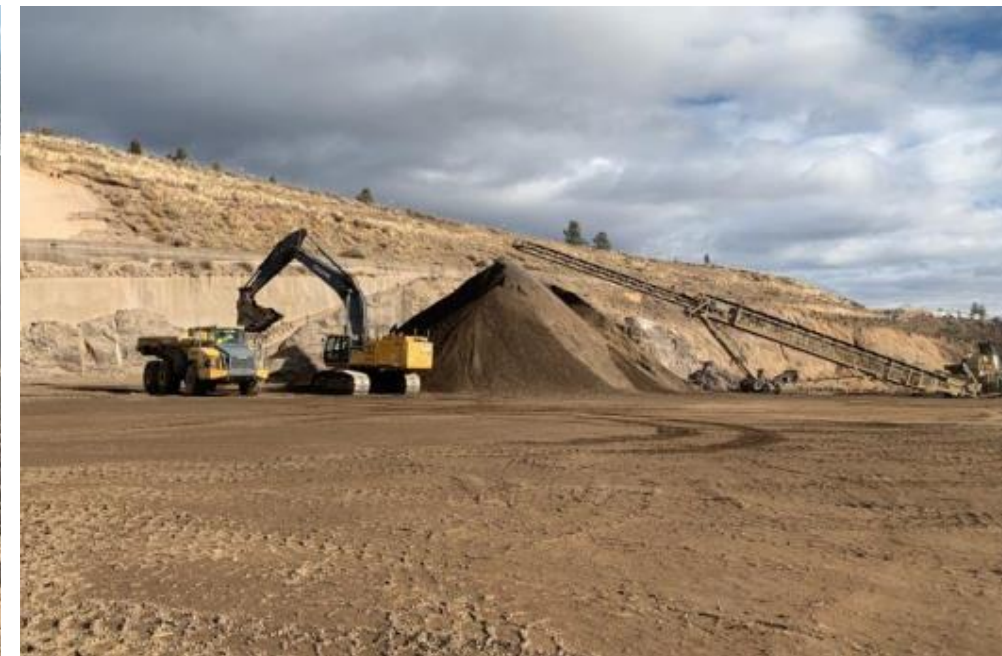
Crusher Stockpiling Material for Pit Floor
