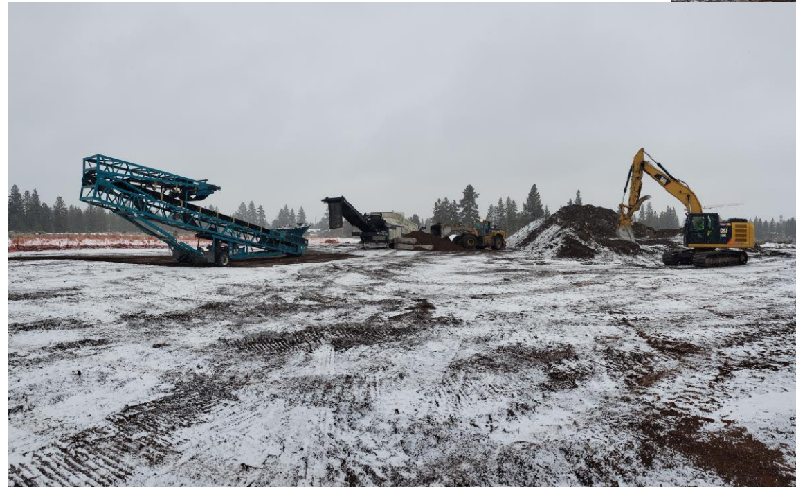
Trommel being setup for screening in Cell 1
