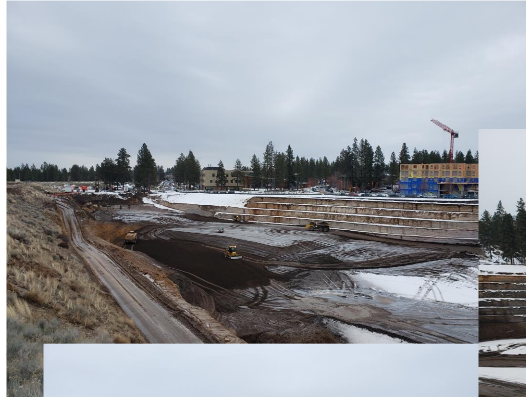
Benching Activities on the north side of the pit
