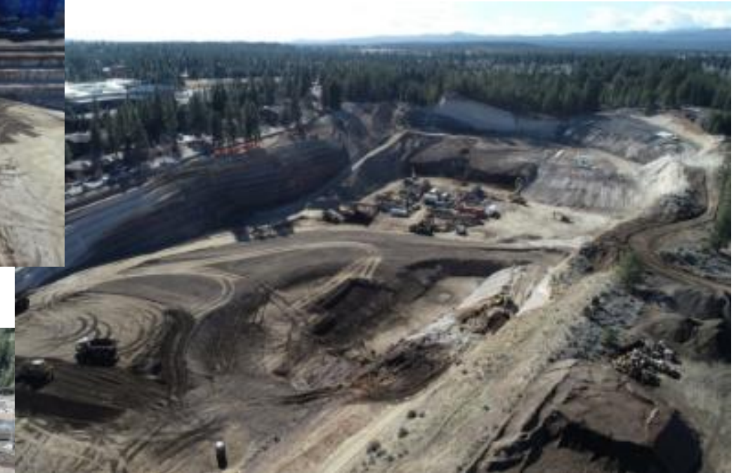
Crushing Activities, Oval Green, and Pit Floor work
