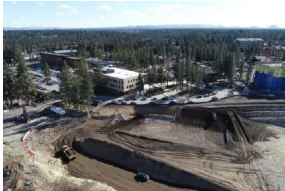
Academic Building 2 – Building Pad Prep
