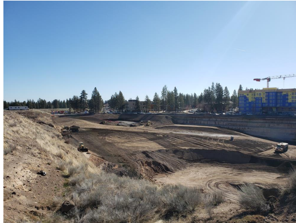
Academic Building 2 – Building Pad Prep and Rock
