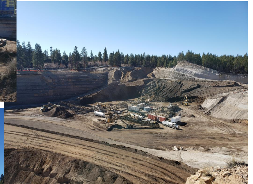
Sloping on the NW side of the pit
