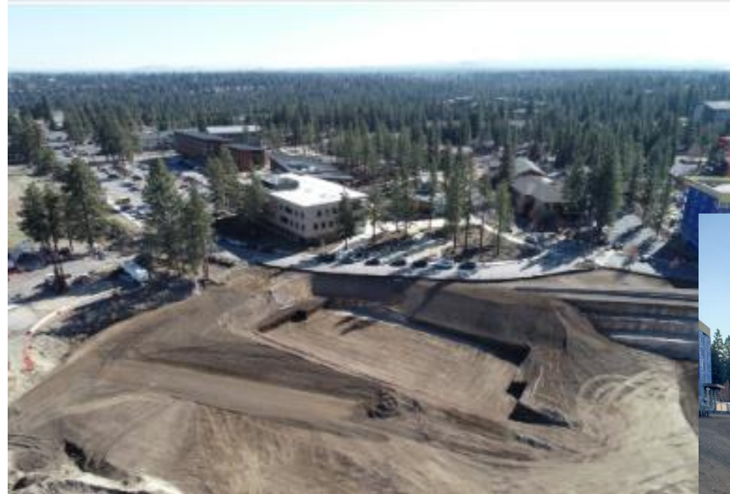
Academic Building 2 – Building Pad Prep
