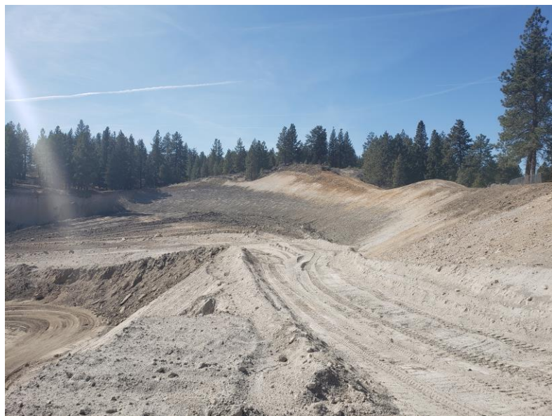
NW Corner of Pit Sloping
