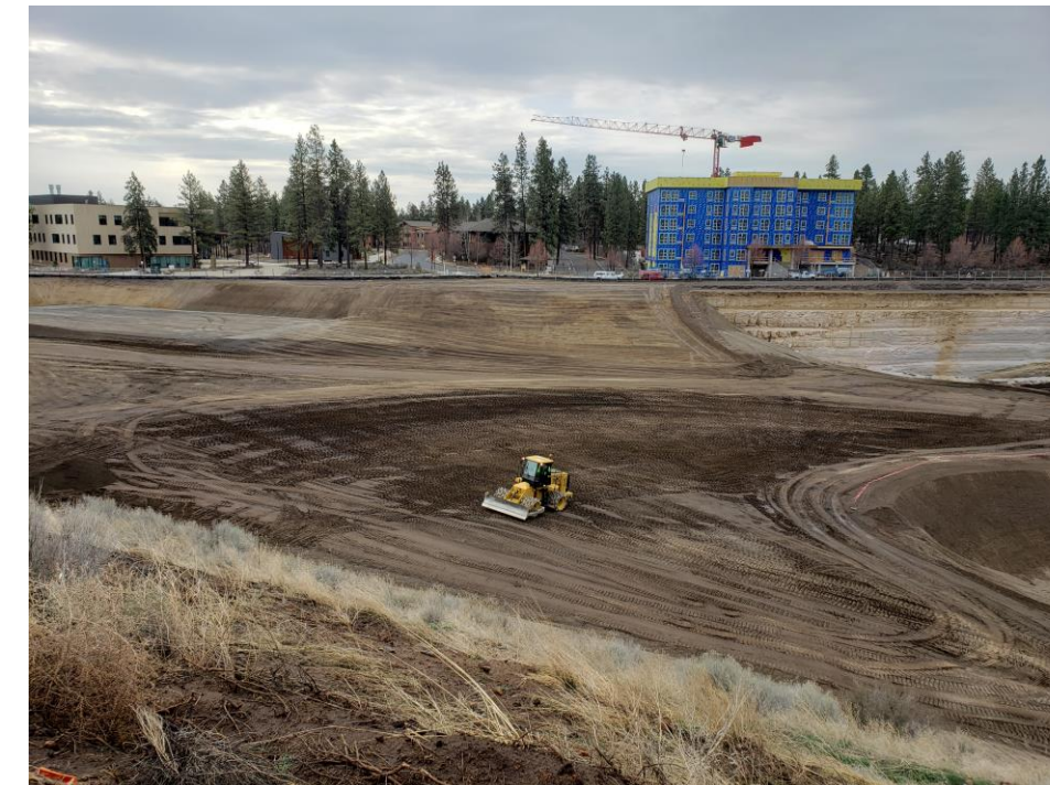
AB2 Rock Pad and South Pit Sloping Activities
