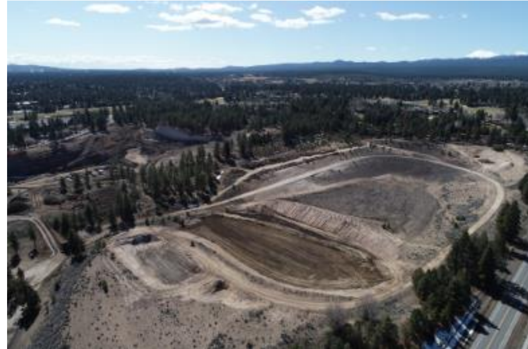
Parking Lot in Cell 3
