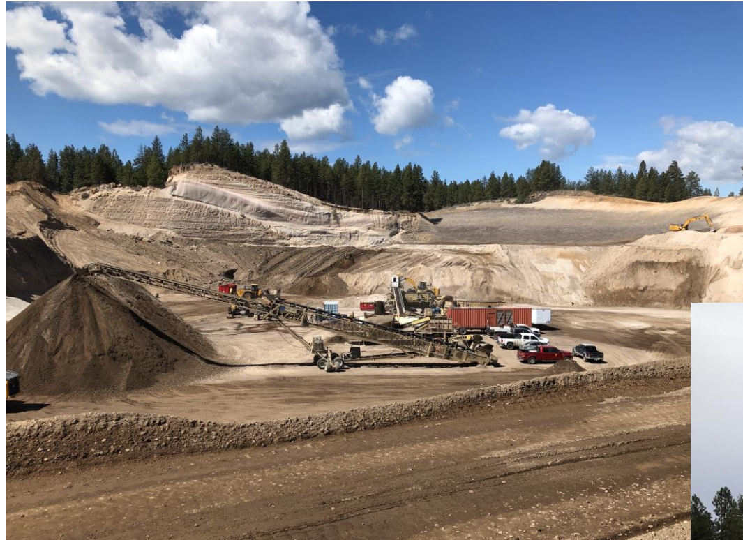
Crushing activities ongoing and SW side of the pit work
