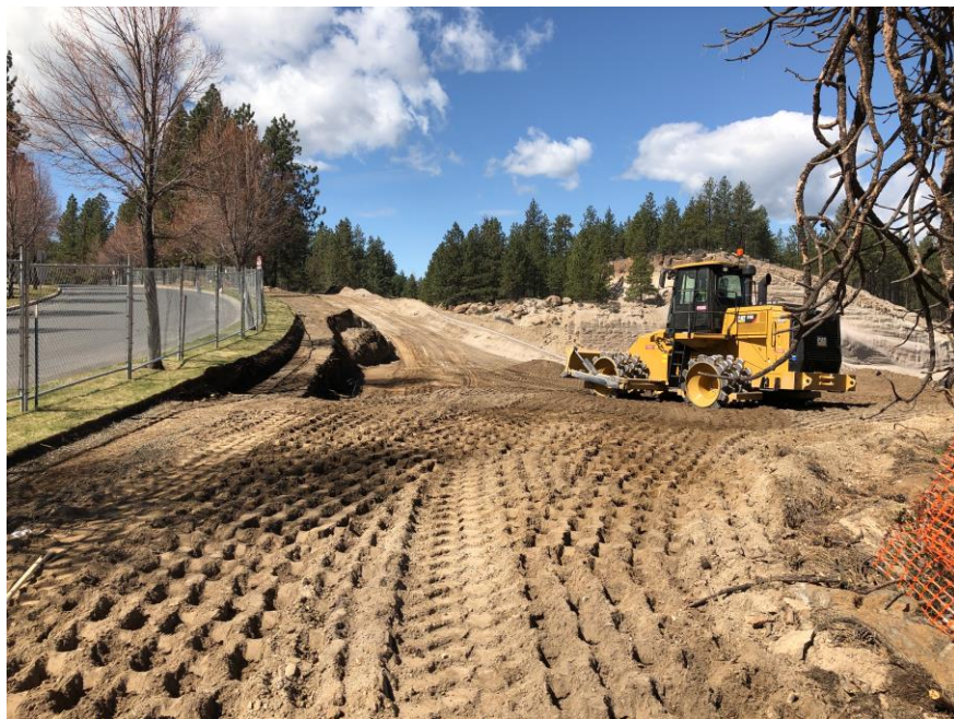
Chandler Sidewalk Grading
