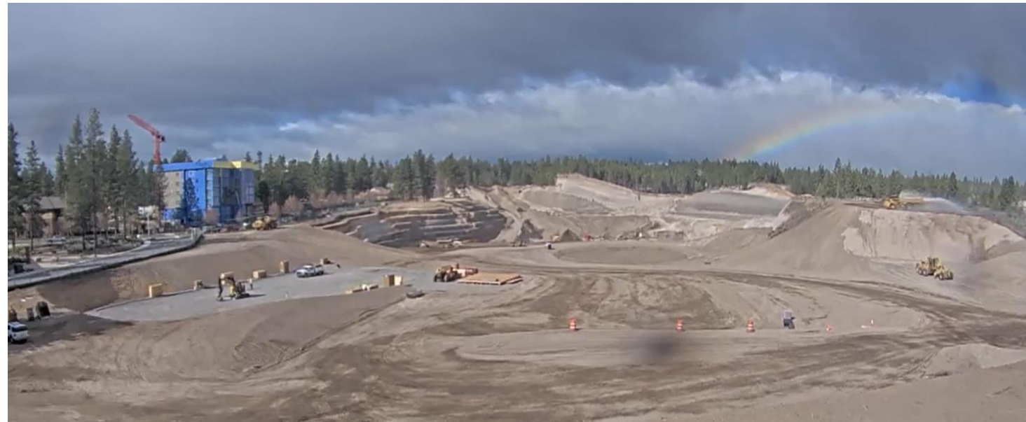
AB2 Pad work beginning, Former Cell 2 work complete
