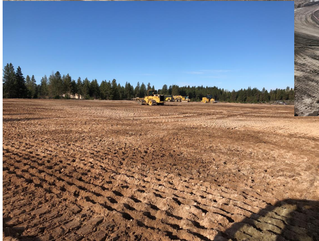
Crushing activities and NW slope of pit
