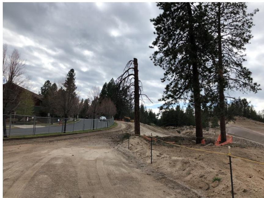
Chandler Sidewalk Grading
