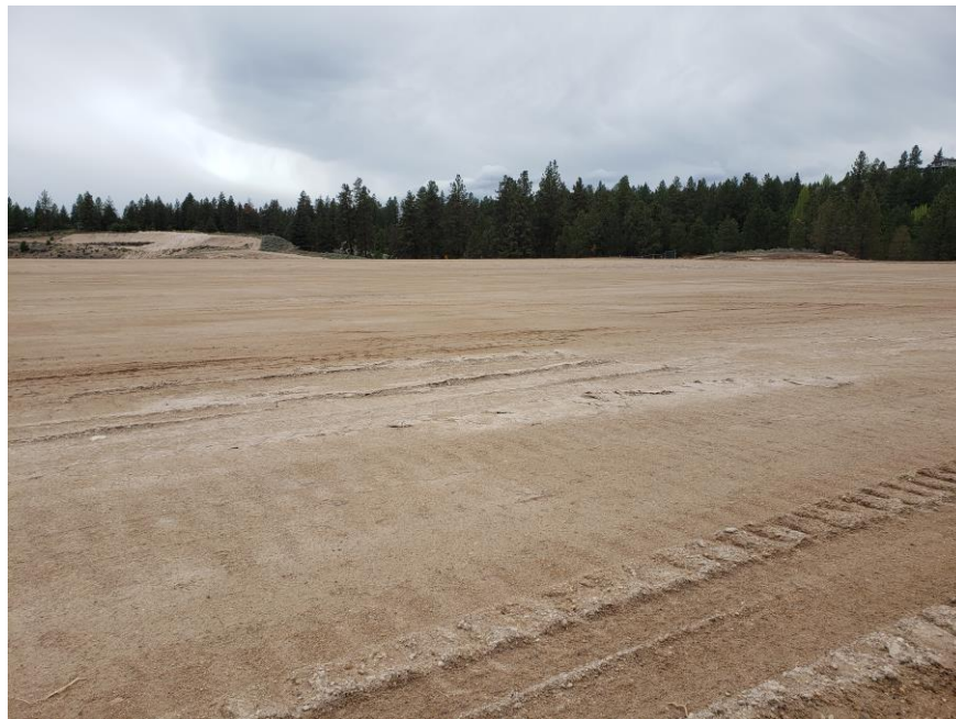
Future Parking lot grading
