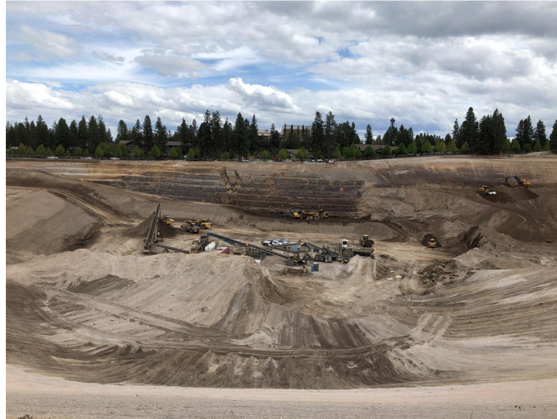
South side of the pit embanking, sloping, and crushing activities
