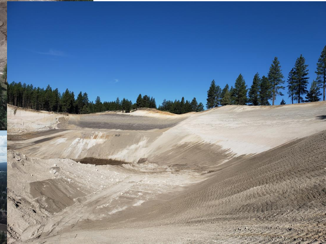
Northwest side of pit sloping
