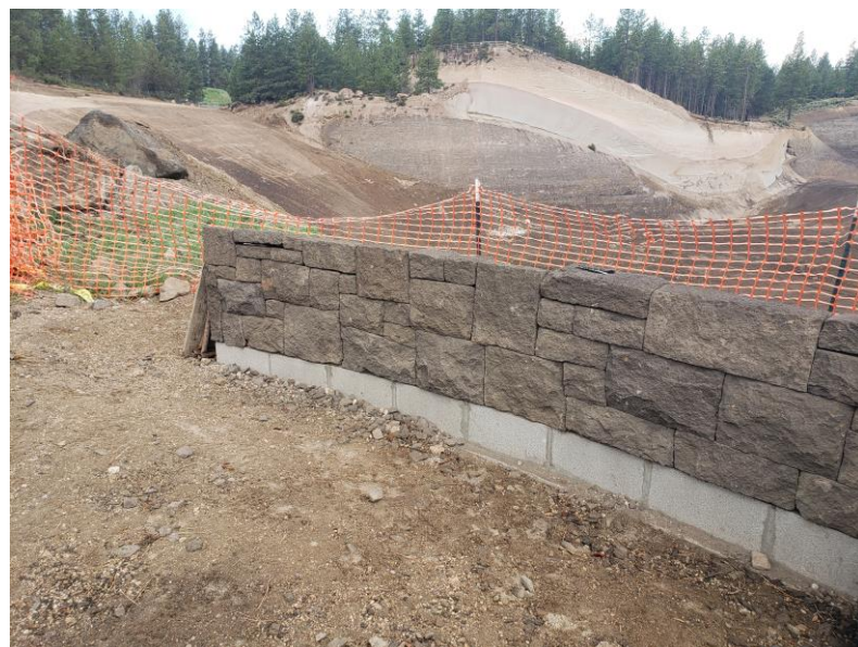
Seat Wall at future Overlook area
