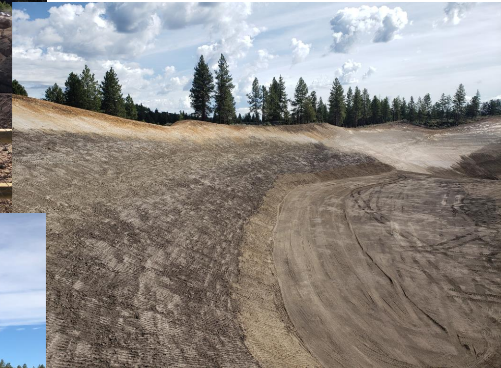
Northwest side of pit sloping
