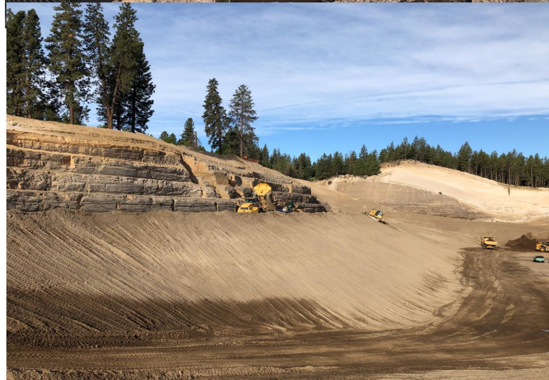
South side of pit embanking and sloping
