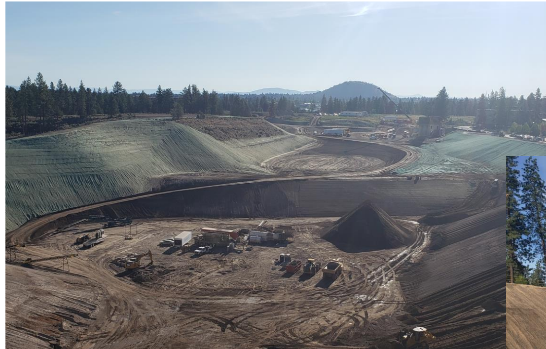
View of the pit looking east – slopes being hydroseeded, oval green complete, and crusher demobilizing
