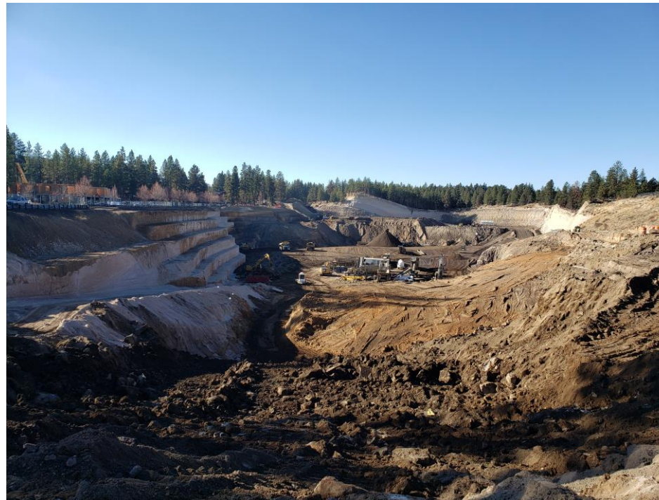
Grading on the east side of the pit floor
