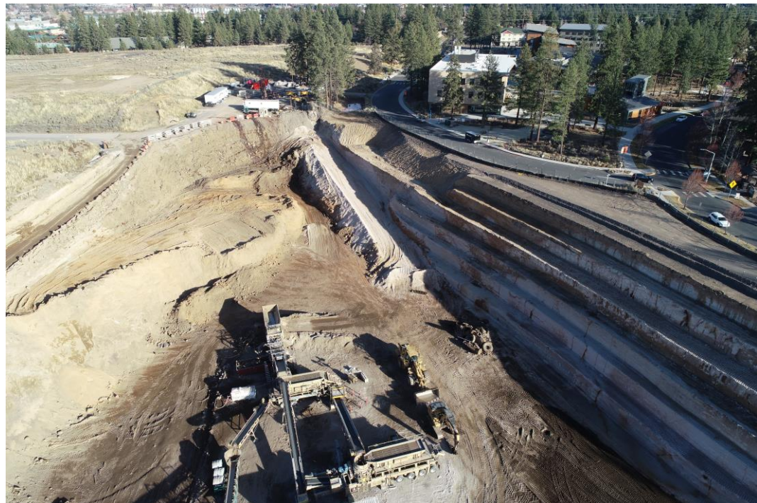
Aerial view of the south benching and Crusher
