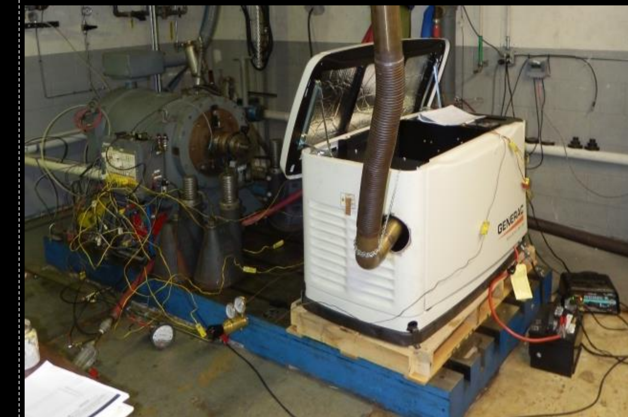
Figure 4 Generac Guardian being instrumented on the test stand at Intertek-Carnot Testing Laboratory in San Antonio, TX.
